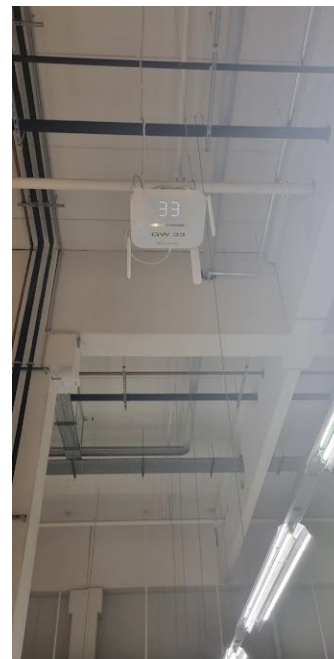
GW is hung lower than surrounding objects and is not close to wall
