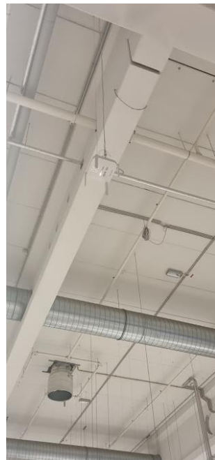
GW is hung lower than the steel beams and no objects are interfering
