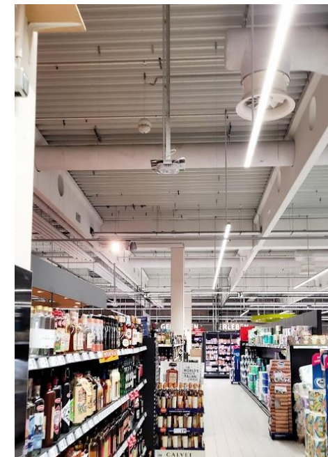
Another good example of a hanging solution. GW is away from near wall and pipes. GW is hung below objects.
